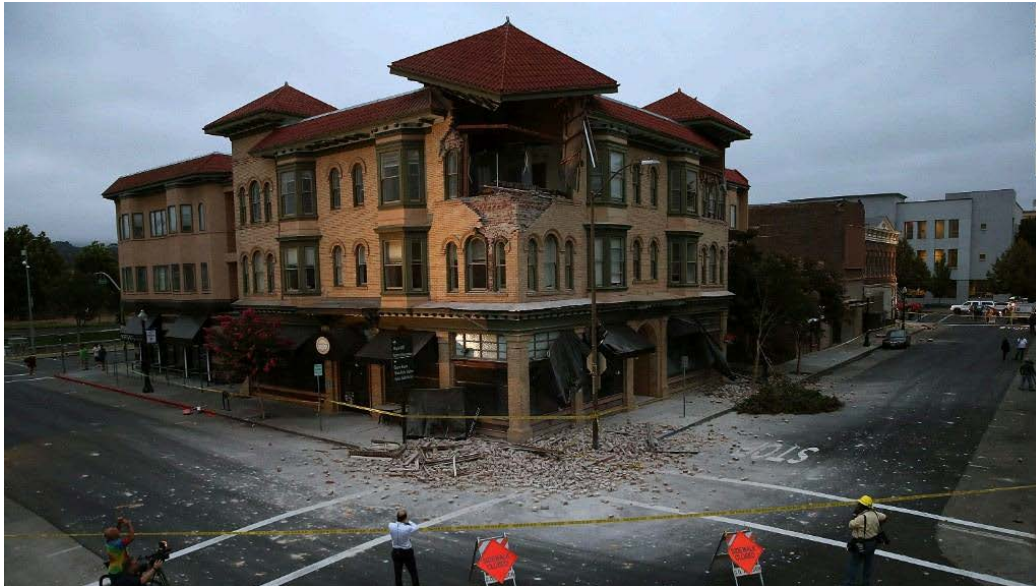
Sunday morning's earthquake jolted Northern California, leaving extensive and widespread damage.
