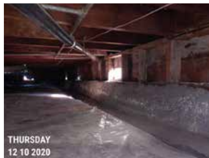
CRAWL SPACE PRE-RETROFIT #2
