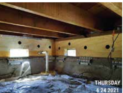
CRAWL SPACE POST-RETROFIT #1
