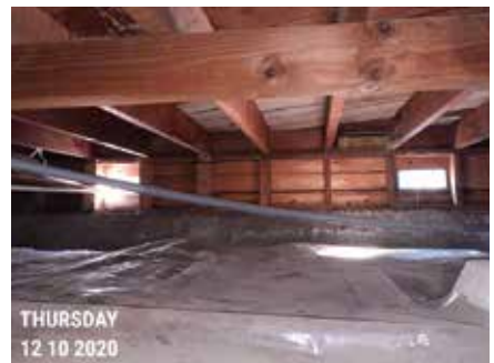
CRAWL SPACE PRE-RETROFIT #3
