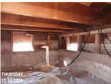
CRAWL SPACE PRE-RETROFIT #1
