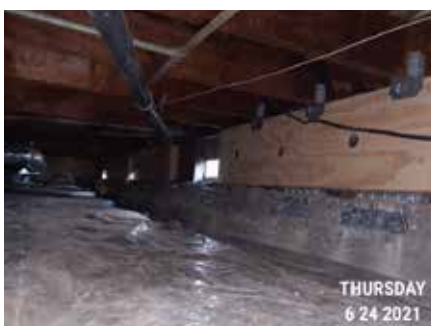
CRAWL SPACE POST-RETROFIT #2
