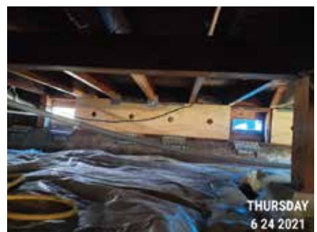
CRAWL SPACE POST-RETROFIT #3
