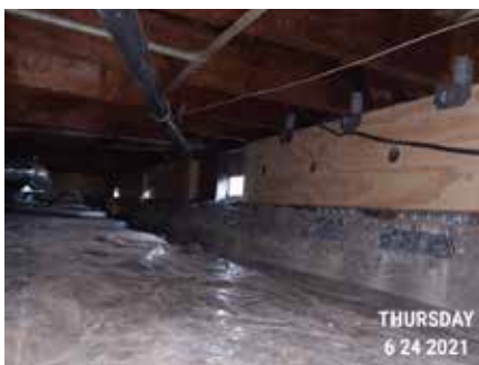
CRAWL SPACE POST-RETROFIT #2
