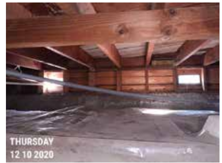
CRAWL SPACE PRE-RETROFIT #3
