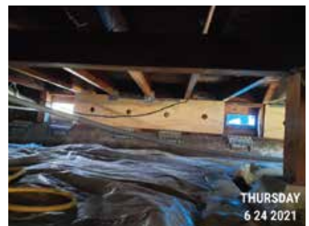
CRAWL SPACE POST-RETROFIT #3
