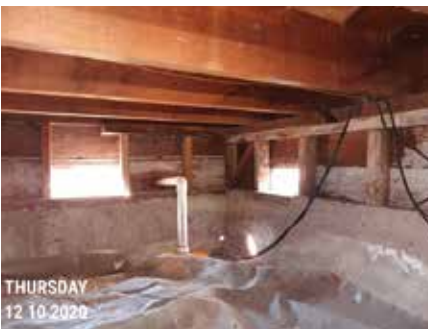
CRAWL SPACE PRE-RETROFIT #1
