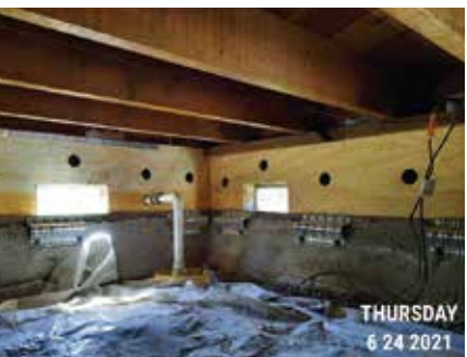
CRAWL SPACE POST-RETROFIT #1
