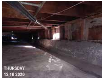
CRAWL SPACE PRE-RETROFIT #2
