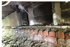
FLOOR-TO-WALL CONNECTION AT PARALLEL JOISTS
